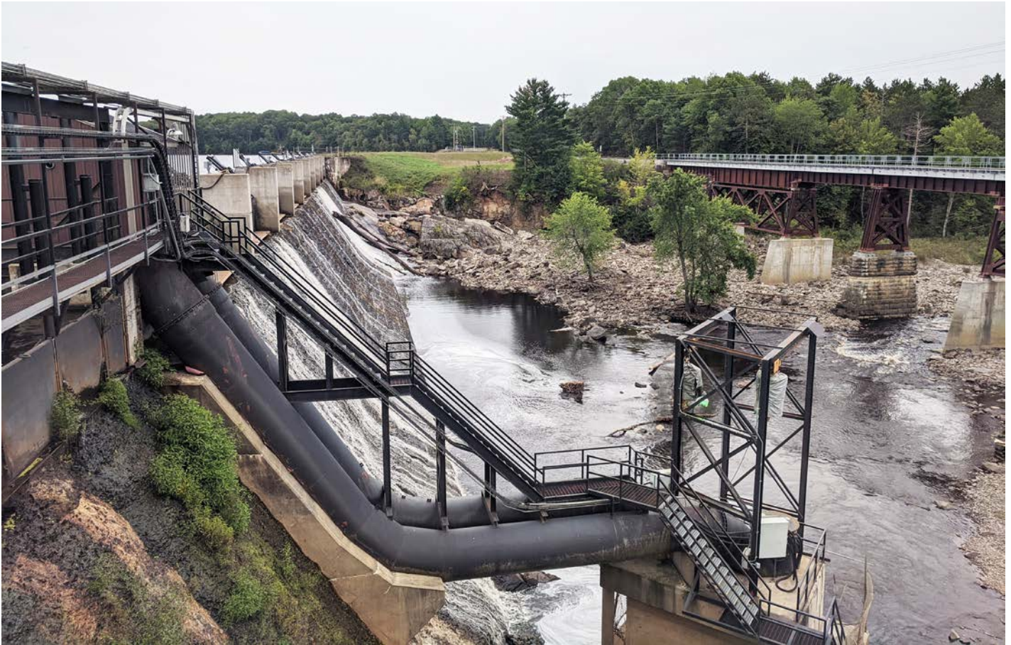
DPO deployed and manages a 1.8 MW bitcoin mining facility at this hydro facility in Hatfield, Wisconsin.
