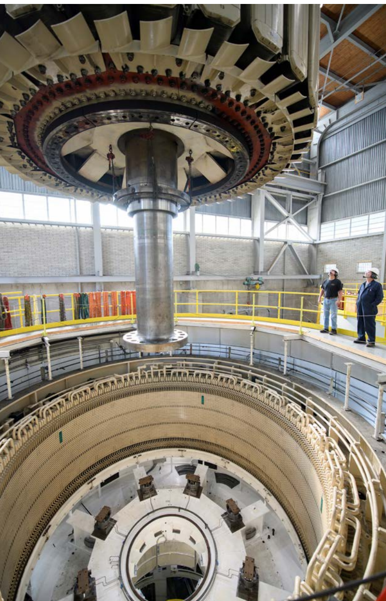
The installation of a rotor at Spring Creek Dam, California, 2024.
