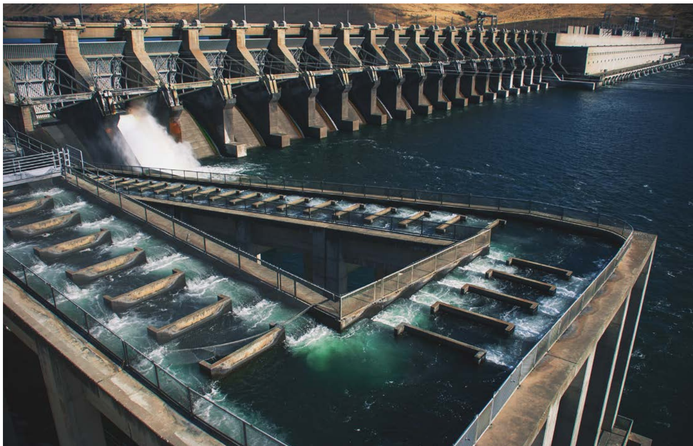
Water flows through the 1,081-foot fish ladder at the Army Corps' John Day Dam, spanning the Columbia River between Washington and Oregon.
