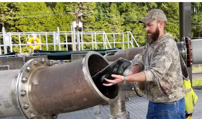
Biologist Brian Wooley releases fish into pipes at Fall Creek Dam that connect to transfer pools where they are then loaded into trucks and safely released back into the wild.
