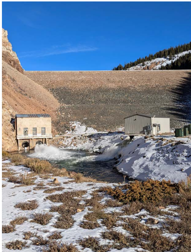
The Taylor River Hydro Project.
