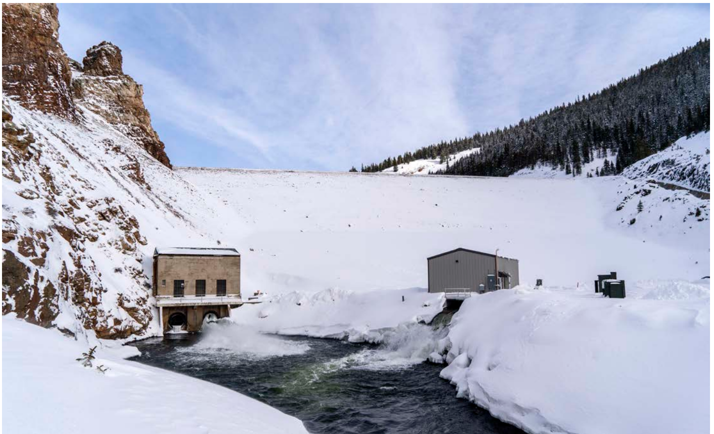
Gunnison County is one of the coldest parts of the country, and in winter, temperatures at the base of Taylor Park Dam can drop to negative 30° or 40° Fahrenheit.
