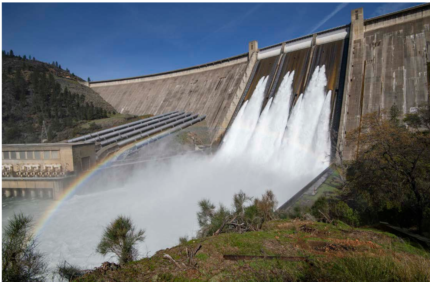
The spillway at Shasta Dam in California.
