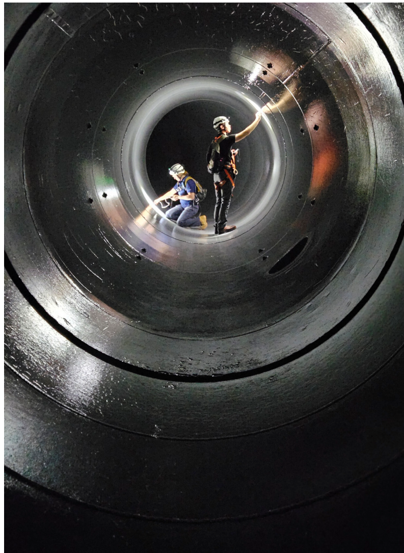
Bobbi Jo Merten and intern Nathan Kral perform final inspection and dry film thickness testing in the lower section of Glen Canyon Dam river outlet works pipe.
