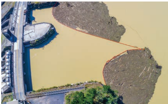
Matahina Dam, NZ during record rainfall event.
