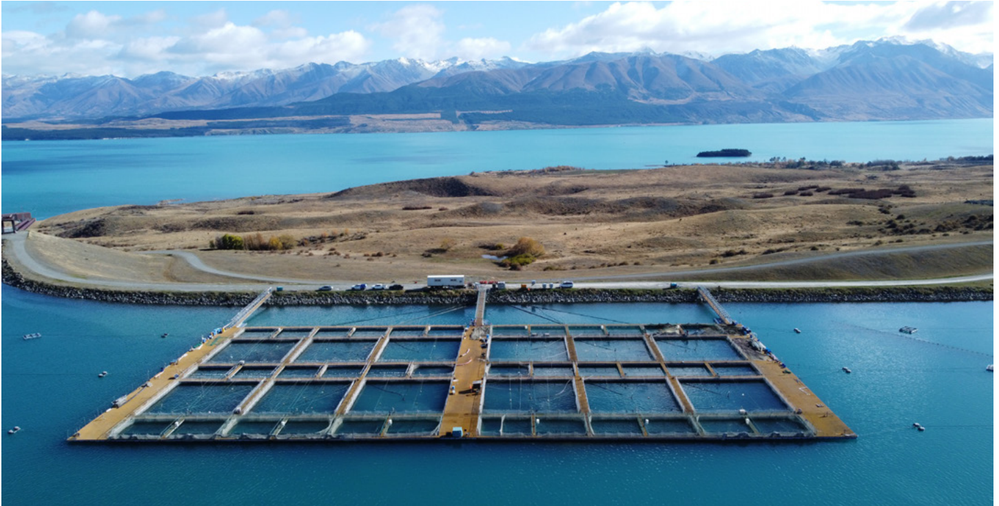
The Mount Cook Alpine Salmon farm at the end of the Tekapo Canal, which links Lake Tekapo with Lake Pukaki, seen in the background. This area is referred to as the stilling basin. There is a major irrigation outlet from the stilling basin that serves a gravity pressure system supplying the Pukaki Flats.
