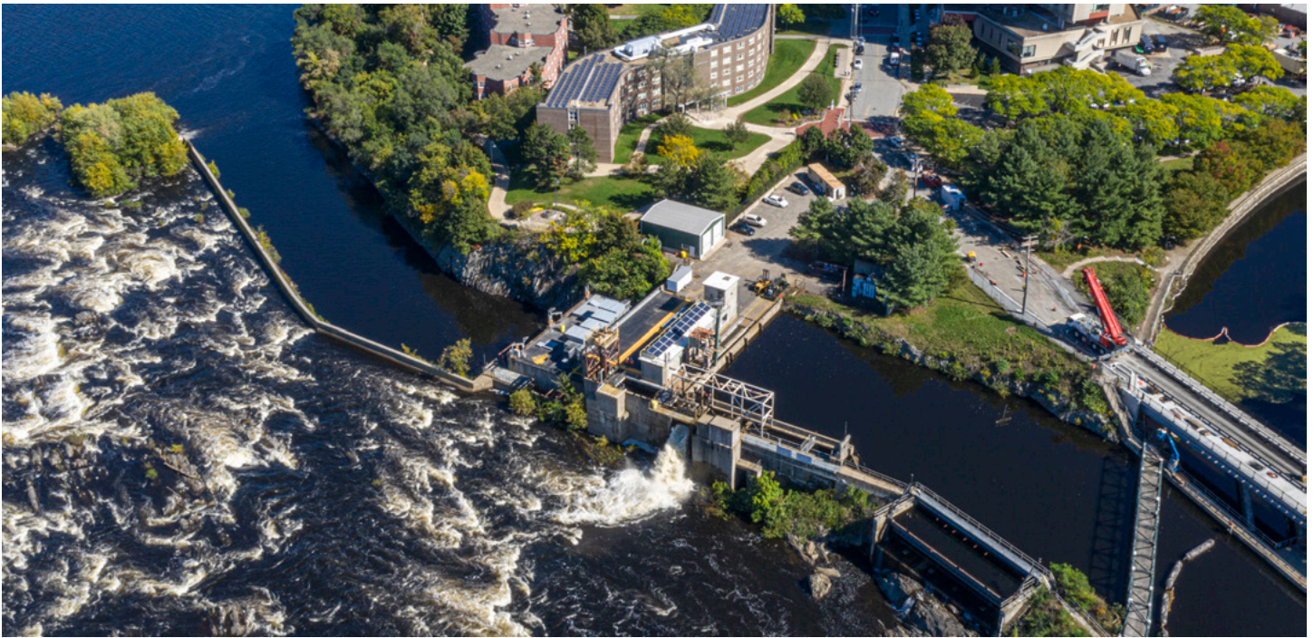
The Lowell Hydroelectric Project, owned by Boott Hydropower LLC, is located in a historic district and is currently pursuing a new FERC license with HDR as its lead consultant.
