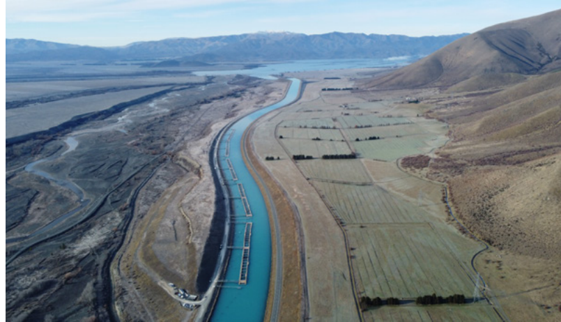
A Mount Cook Alpine Salmon farm in the Ohau C Canal, located alongside some of the early border-dike irrigation carried out by Glencairn Station with water supplied by siphon from the canal. Visible along the right side of the photo is a headrace against the foothills that is supplied from the Ohau B Power Station intake.
