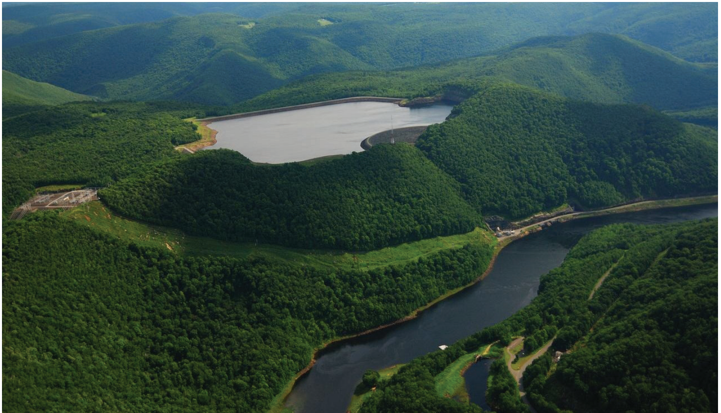
In addition to supporting dam safety and engineering work, HDR is the lead consultant for the relicensing of Brookfield Renewable's Bear Swamp Pumped Storage Project.
