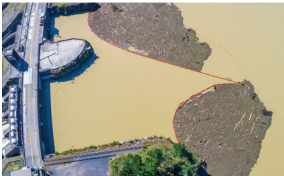
Matahina Dam, NZ during record rainfall event.
