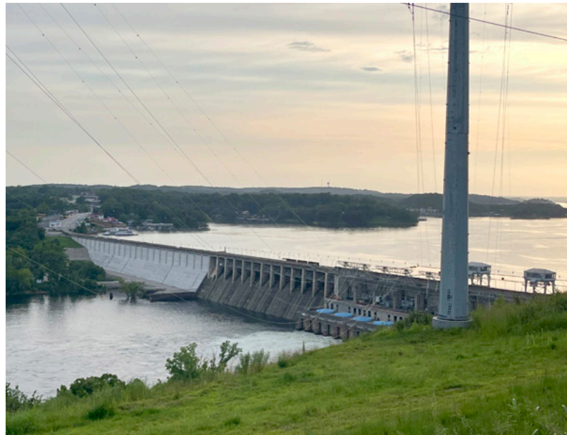
A photo taken during a daily inspection of the Osage Hydroelectric Project in Missouri, conducted by GZA and the site operator in support of the external owner's dam safety program.
