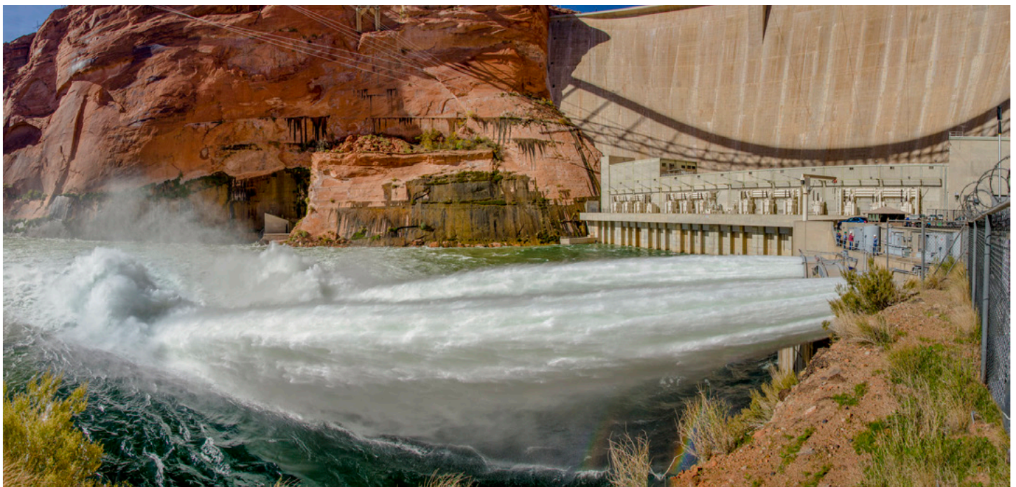
A high-flow experiment at Glen Canyon Dam in 2018, designed to rebuild sandbars.
