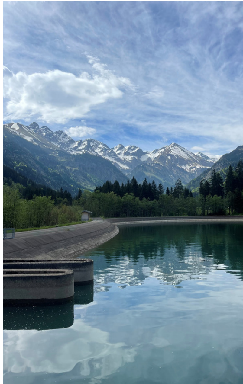
The Warmatsgund hydroelectric plant in Oberstdorf, Germany, uses HYDROGRID Insight.
