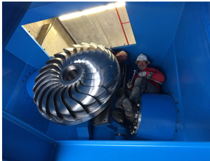
A new Turgo runner is installed at Powerhouse 2 in 2015.
