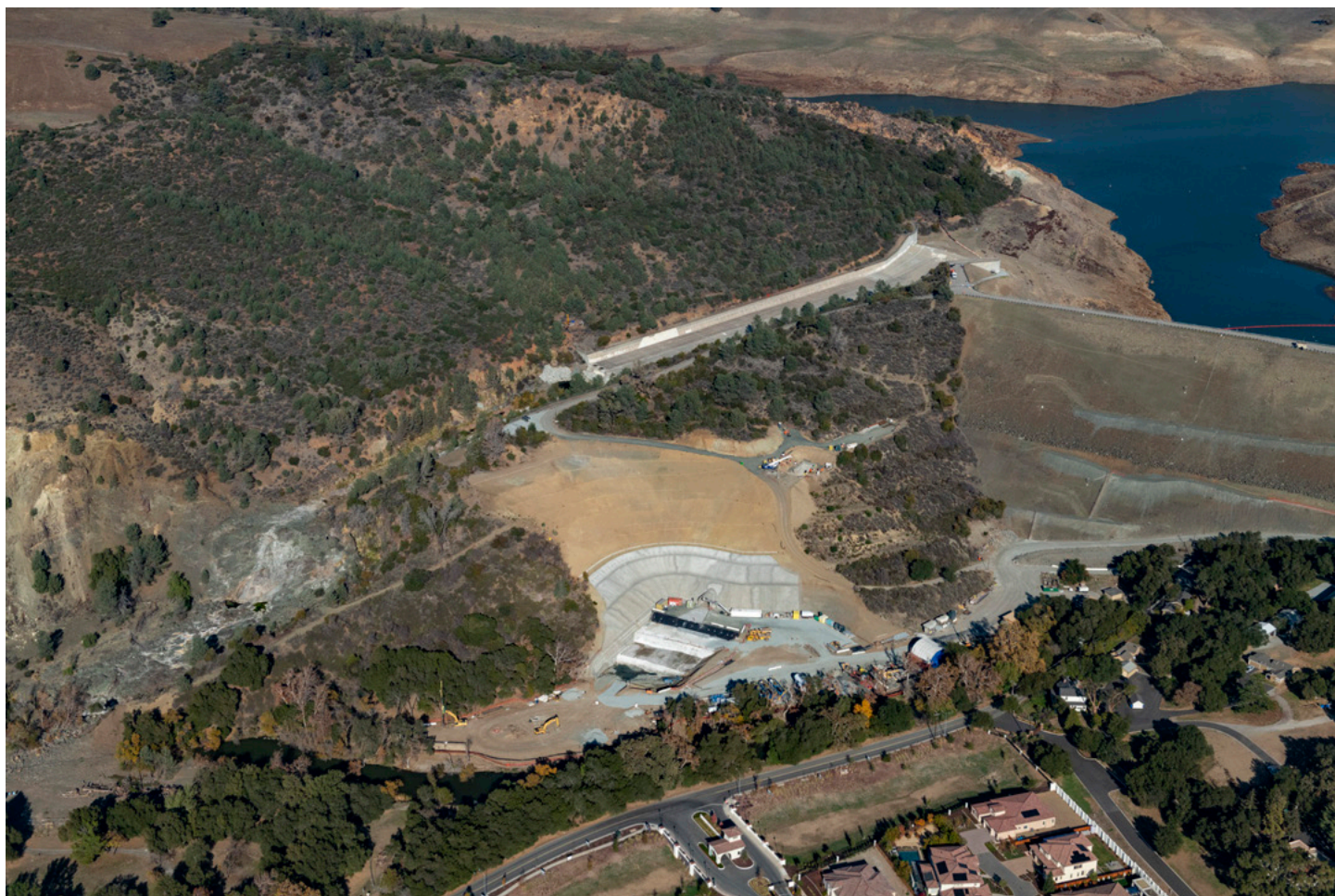
Santa Clara Valley Water District's Anderson Dam Tunnel Project includes the construction of a new low-level outlet system consisting of a 1,700-foot tunnel up to 24 feet in diameter. The project is part of the larger upcoming Anderson Dam Seismic Rehabilitation Project, estimated at over $1 billion, which will include the seismic rehabilitation of the 235-foot-high dam, the construction of a new spillway, and the completion of the outlet system.
