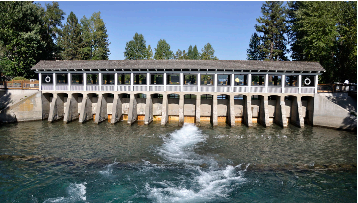
Reclamation modified the 109-foot-long Lake Tahoe Dam in 1987 under the Safety of Dams program.
