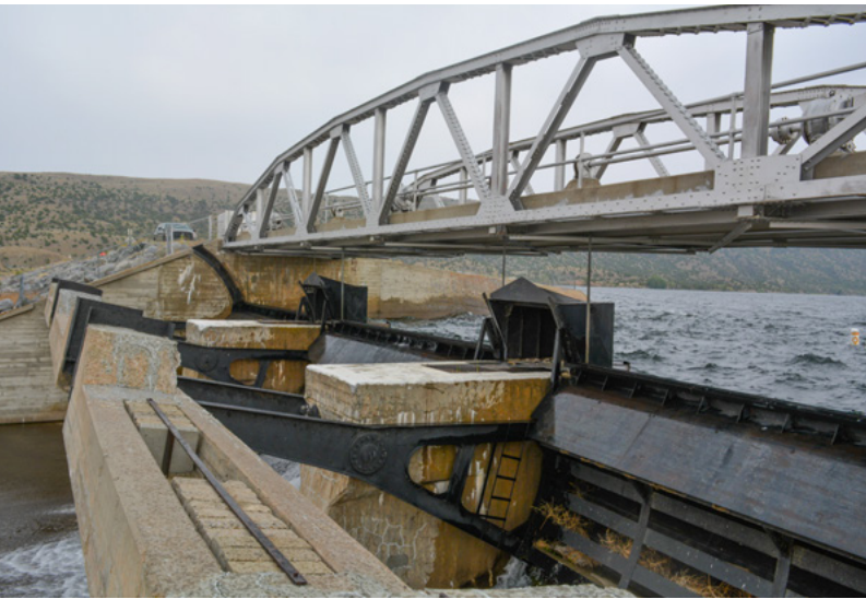
Spillway gates at Bull Lake Dam in Wyoming.
