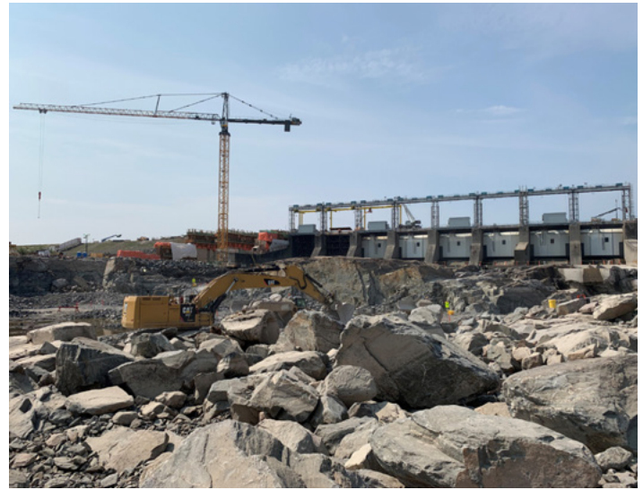
Another view of work on the Little Long Dam safety project.
