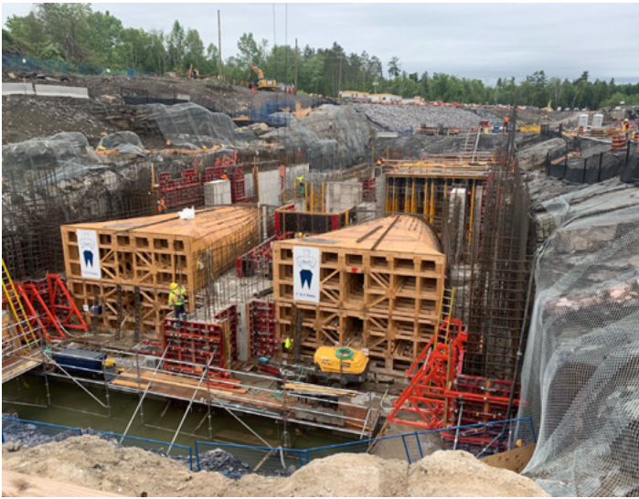
Work on the Little Long Dam safety project.
