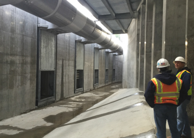
ISI's largest hydro facility screen install, a 550 cfs Pacific Gas & Electric structure on the Stanislaus River in California.
