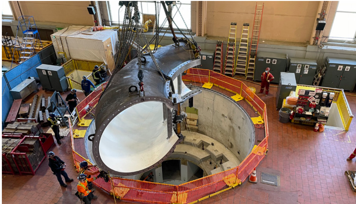
The replacement of a scroll case at the Adam Beck I Generating Station in Niagara Falls.
